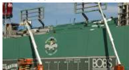
INSTALLING GREEN MONSTER SEATS
