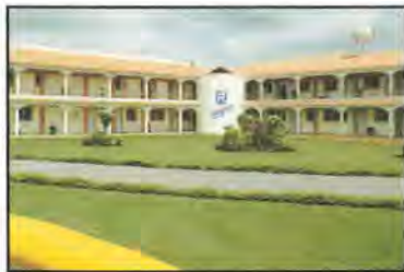
Housing and office facilities at Royals Dominican complex
