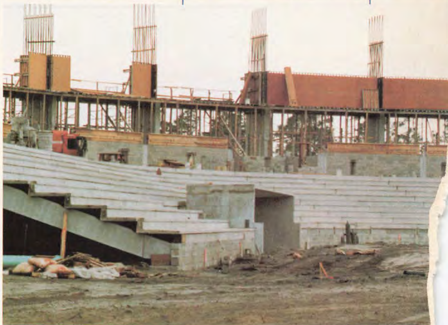
Construction is underway for the 1988 New York Mets training stadium.
