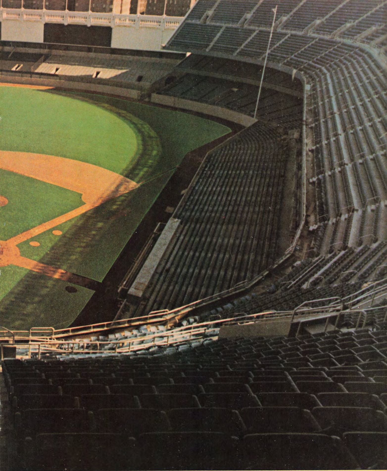
a singularly unique structure, recognizable even in its new form to any baseball fan.
