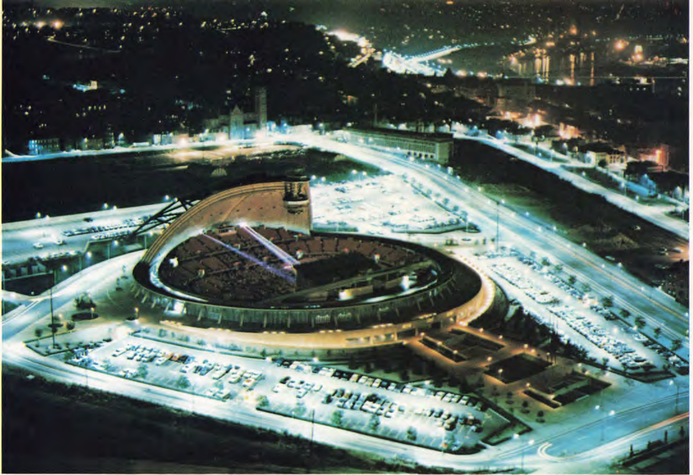
Civic Arena with roof open (above), view from new U.S Steel Building (below).
