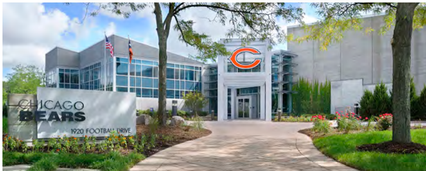
New west addition to Halas Hall along with a new entry canopy leading to the main lobby.
