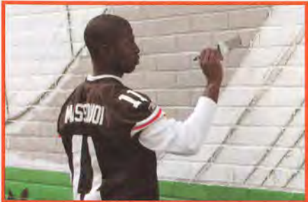
Wide receiver Mohamed Massaquoi helps paint during the installation of an outdoor fitness zone at Famicos Foundation Park Village Apartments in Cleveland.
