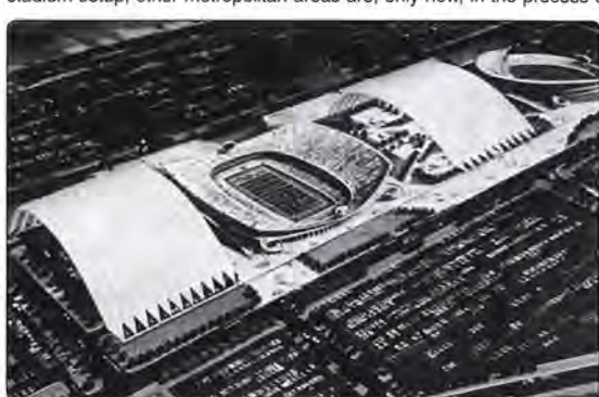
Original plans for the Truman Sports Complex called for a rolling roof which could cover Arrowhead or its baseball counterpart, Kauffman Stadium - a revolutionary concept at the time.
