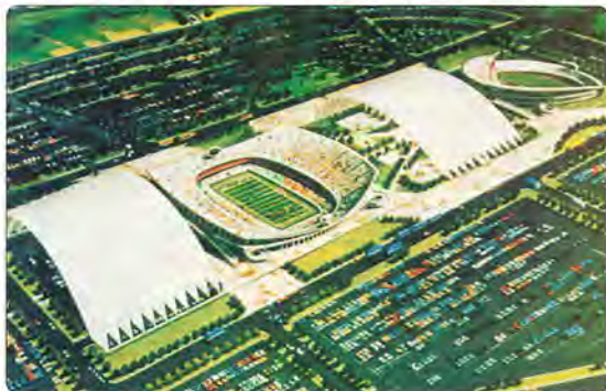
Original plans for the Truman Sports Complex called for a rolling roof which could cover Arrowhead or its baseball counterpart, Kauffman Stadium - a revolutionary concept at the time.
