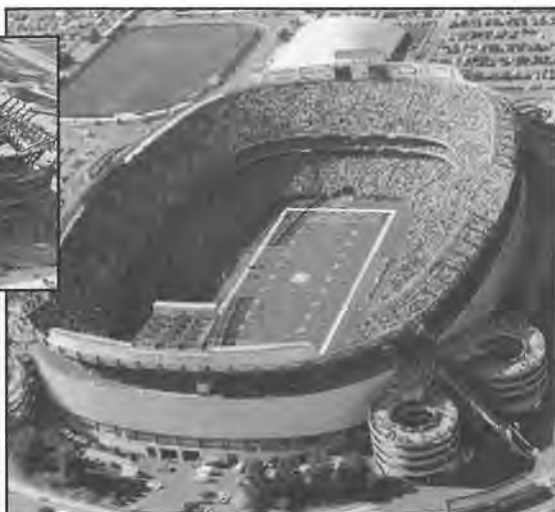
GIANTS STADIUM (WITH INDOOR AND OUTDOOR PRACTICE FACILITIES IN THE BACKGROUND).
